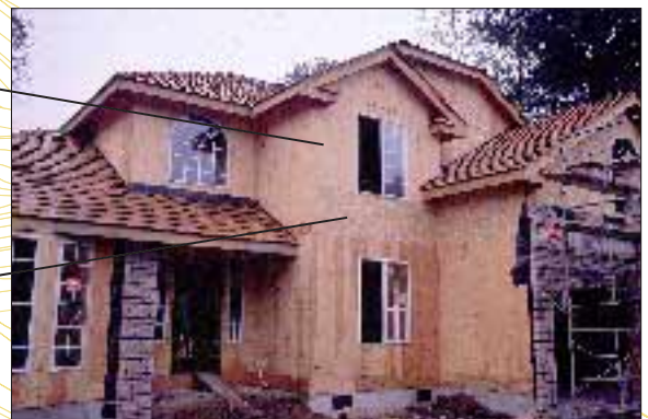
Structural Panels in their construction application.
